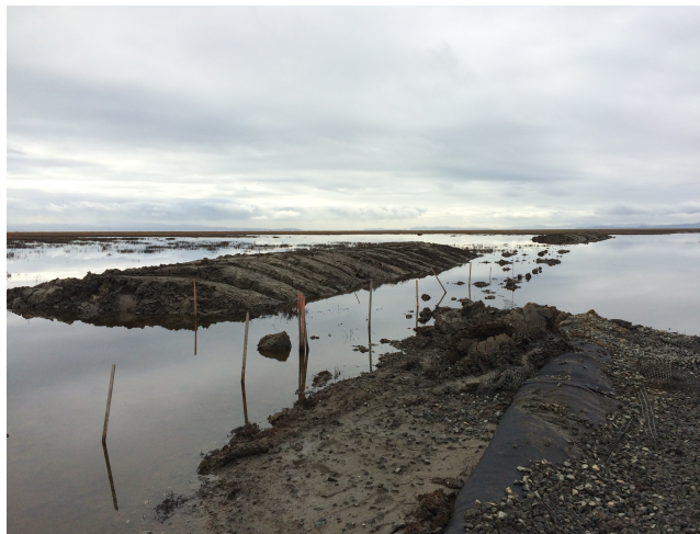
Figure 17. Marsh mounds will provide habitat for wildlife in high tide events. The channel, to the right of the two pictured marsh mounds, cannot be seen in these high tide events.
